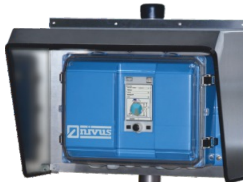
Field enclosure installation
